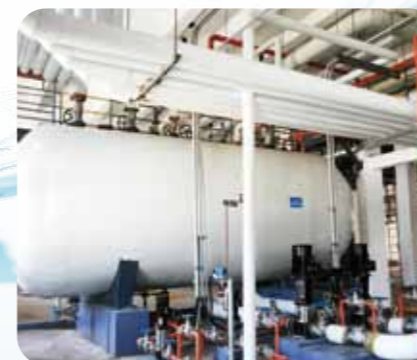
Condensate polishing treatment filtration in Power Plant
